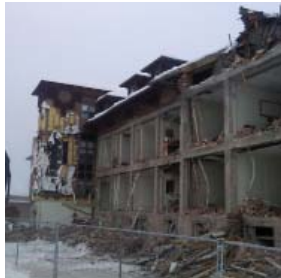
Mills Hall demolition; Helena, Lewis & Clark County
