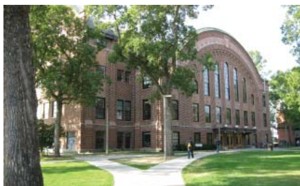
Romney Gym; MSU Bozeman, Gallatin County
