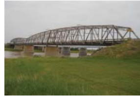
Yellowstone River Bridge at Fallon; Prairie County
