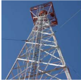
McDonald Pass Airway Beacon; Powell County
